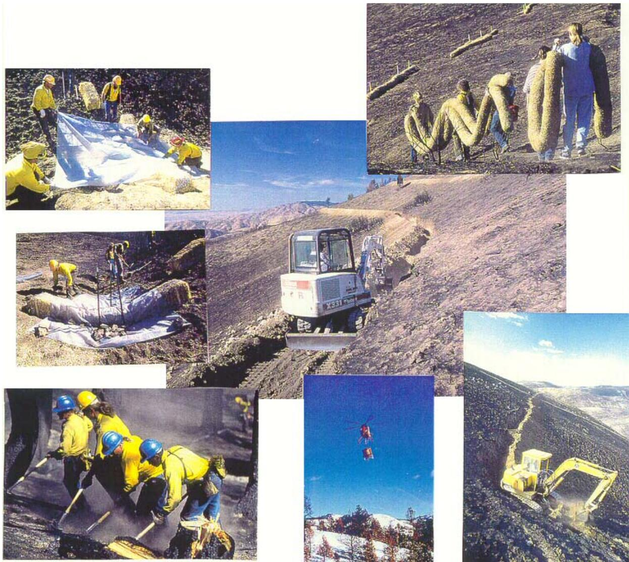
Figure 3. Examples of BAER treatments (Clockwise from the upper right): Straw awattle placement, terrace construction, contour trenching, aerial seeding, log erosion barrier placement, straw wattle dam installation, and streambank armoring.
